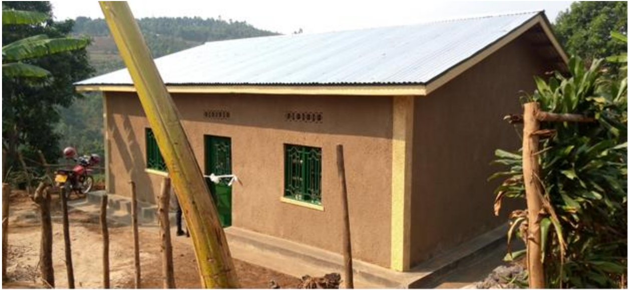
Inauguration Ceremony of the house constructed in Cyangugu Zone
